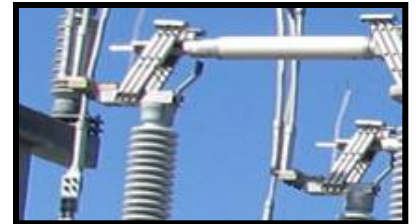
SUBSTATION CONNECTORS
